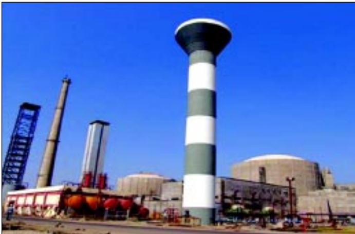
Tarapur Atomic Power Project-3
