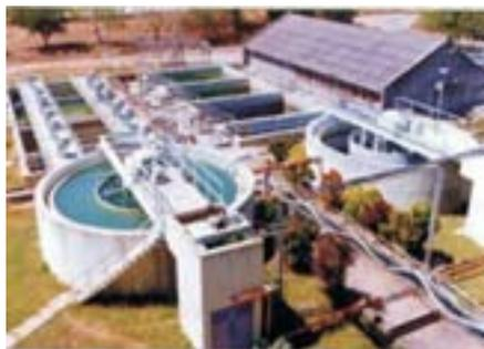
Low level waste treatment by chemical precipitation at Centralised Waste Management Facility, Kalpakkam
