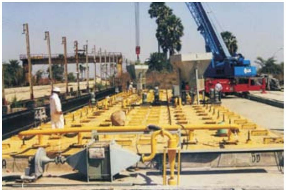
*In-situ solidification in Reinforced Concrete Trenches*
