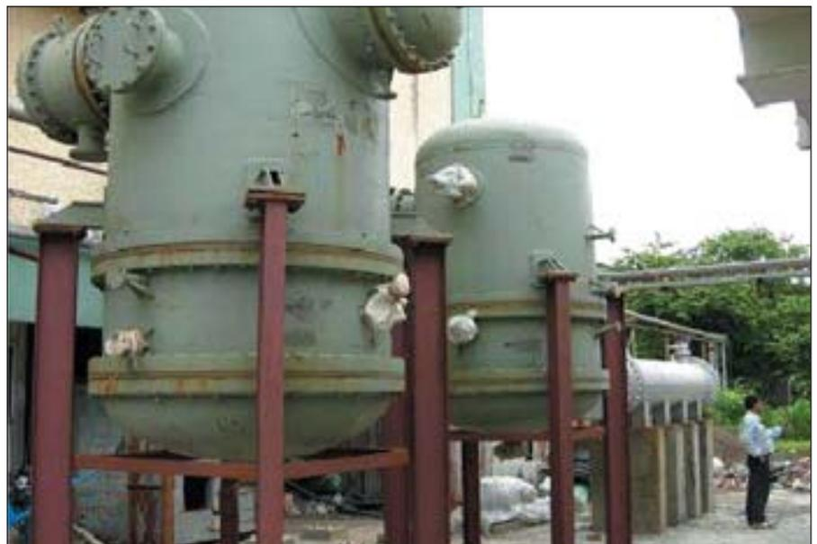
Fig. 2: 50,000 litres/day 2-Effect LTE Desalination Plant (under installation)
