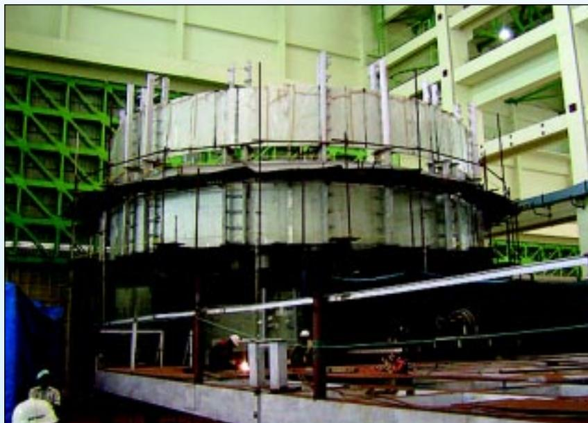
*PFBR Safety vessel fabrication under progress*
