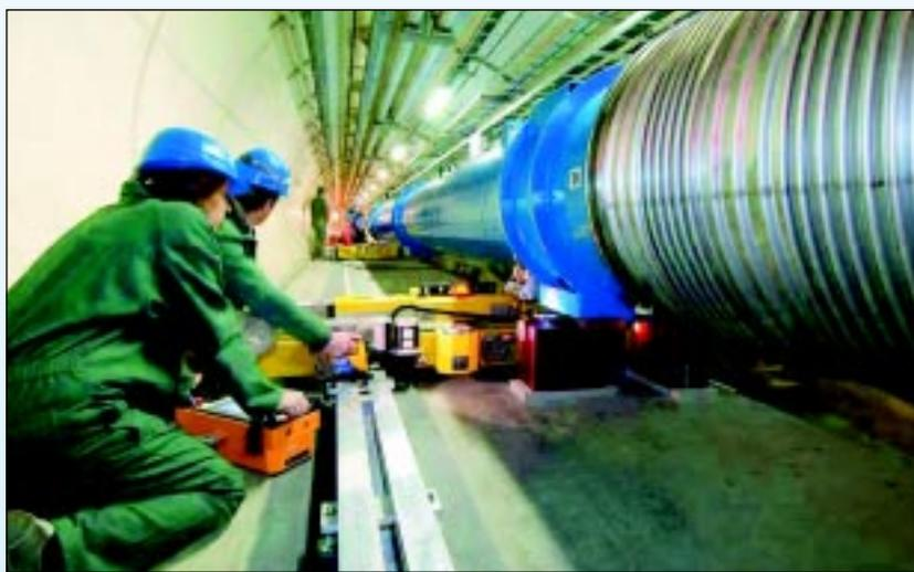
*Dipole assembly weighing 32 tons being installed on jacks supplied by Raja Ramanna Centre for Advanced Technology for the Large Hadron Collider at CERN, Geneva*
