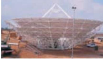
(BARC) and Electronics Corporation of India Limited (ECIL) develop a 32 metre diameter Indian Deep Space Antenna System – IDSN 32 for providing steering, tracking and science data reception support for ISRO's Moon Mission – Chandrayaan-I.
